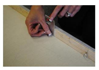
3. Attach the panel using the 2 supplied screws. Repeat for other bracket.
